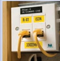
Telephone and Network faceplates
